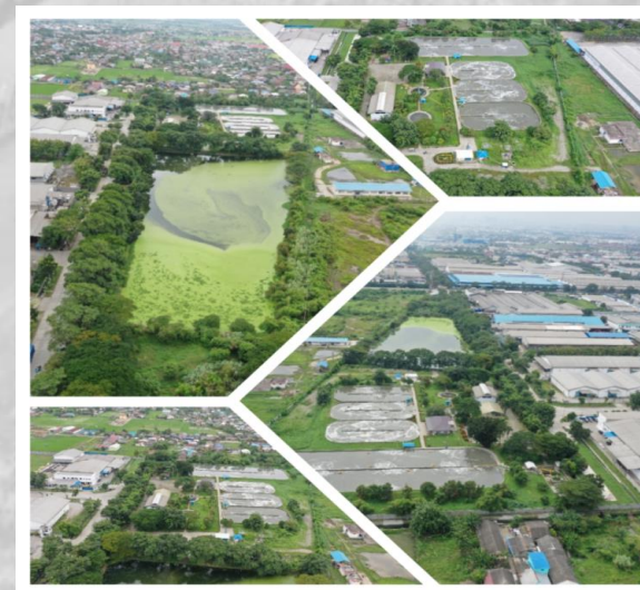
Waste Water Treatment Facilities PT Kawasan Industri Medan Capacity 21.600 M3/Day
